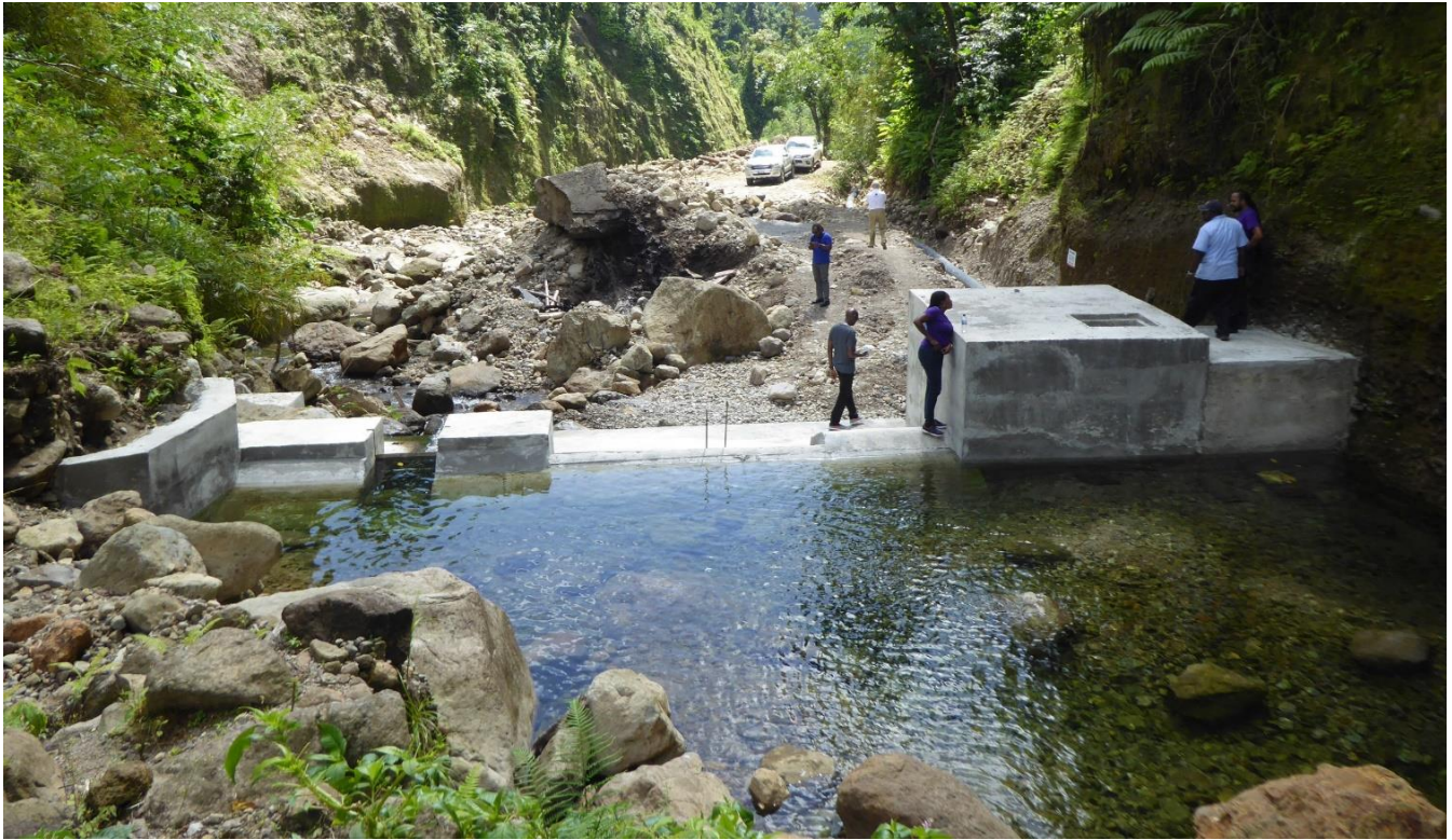
Water intake in Dominica under reconstruction using a more resilient design in following its destruction during flooding caused by Hurricane Maria in 2018.
