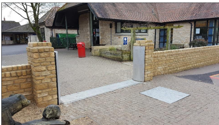
Self-activating flood gate (gate rises itself when floodwater enters underground control chambers)
