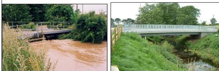
Old culvert in Romanby replaced with a new bridge to improve through-flow and reduce upstream water levels without detriment to designated flood zones downstream
