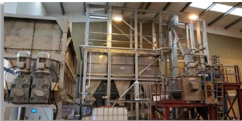
CCm Technologies' full-scale demonstration plant
