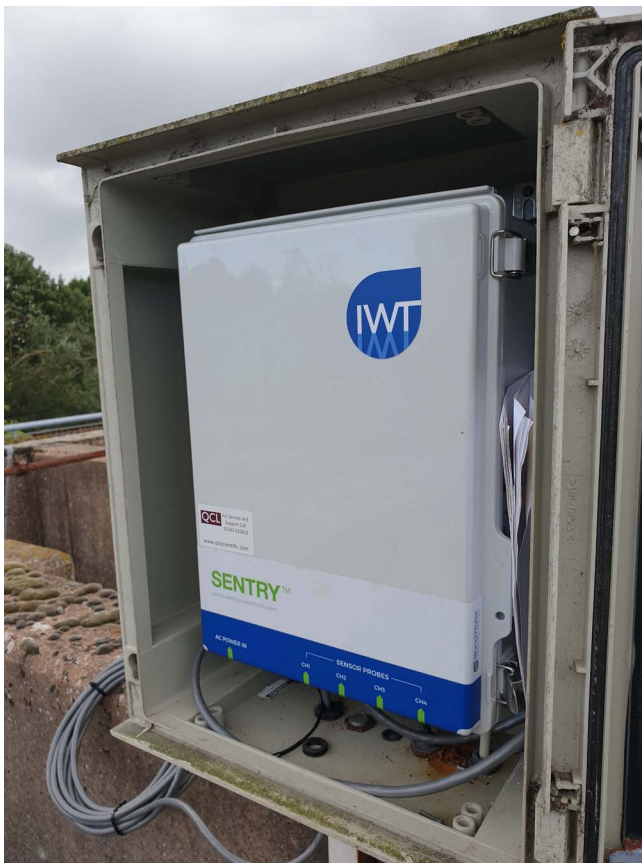
Figure 2: SENTRY control system installed at the Wessex Water, Site A, WWTP.
