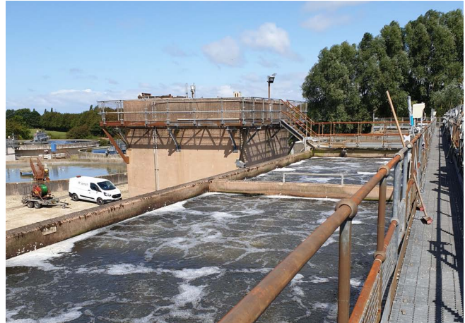
Figure 1: SENTRY sensors installed upstream of the Biologically Aerated Flooded Filter
