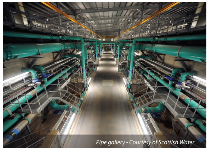
Construction is underway - Courtesy of Scottish Water
