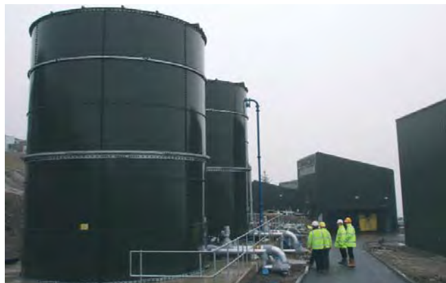
Sludge Holding Tanks
