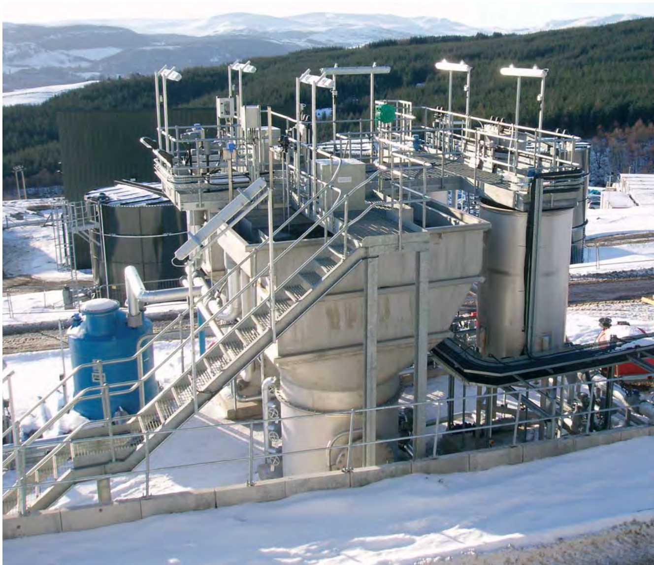
Multiflo Sludge Plant
