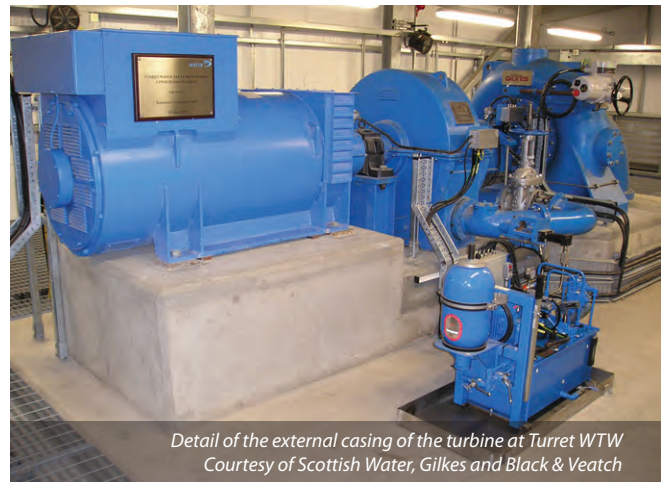
A Gilkes turbine installed at a WTW by Black & Veatch Courtesy of Scottish Water, Gilkes and Black & Veatch
