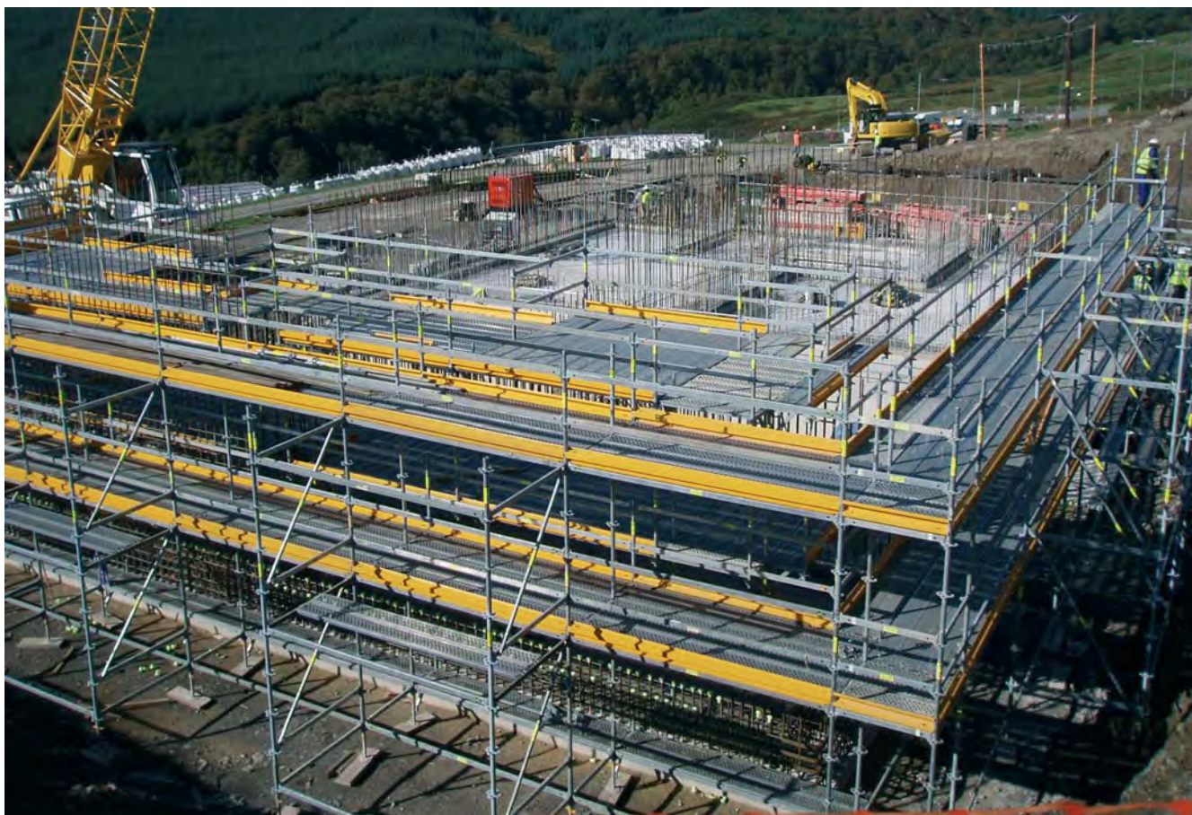
Chlorine Contact Tank
