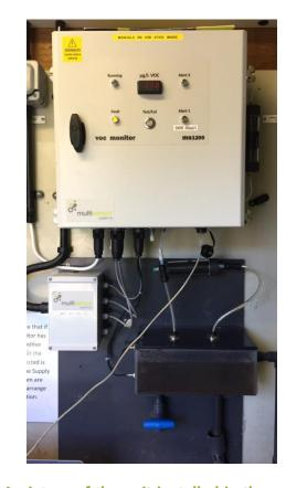
A picture of the unit installed in the outbuilding. The unit controls a sluice gate which diverts flow away from the reservoir in the event of contamination.
