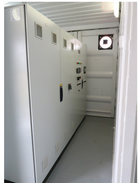
Containerised Control Panels
