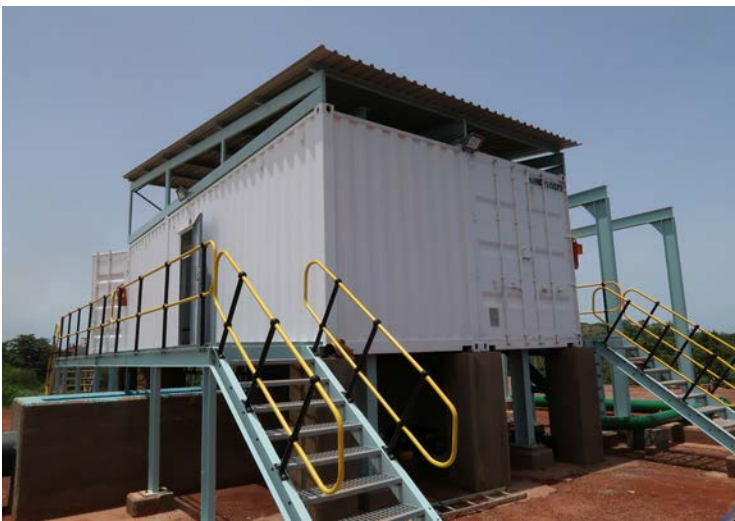
Containerised Powerhouse
